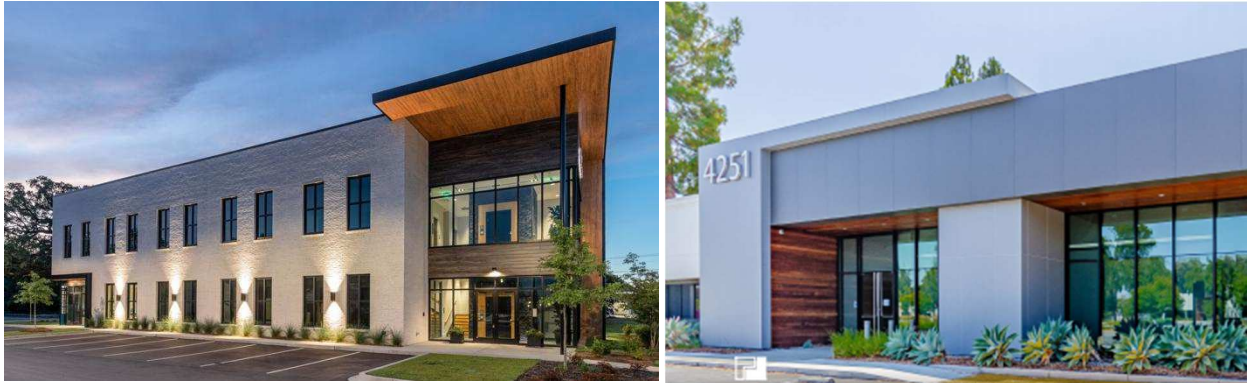
Representative one-two storey office building facades.
